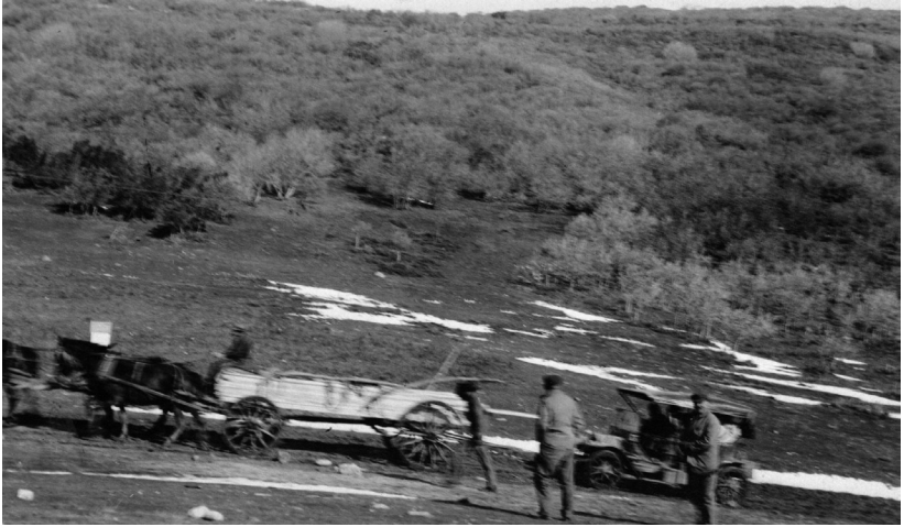
#5 (Bottom left) "Along the road east of Evanston Wyo" Evanston is on the western edge of Wyoming with Utah just across the border.
