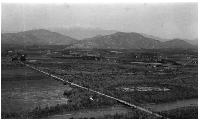
#31 "Looking north from Mt Roubidoux" The steel bridge across the Santa Ana River, shown here, was washed out in 1916. Following the road (today's Mission Blvd.) to the middle left side there are two groups of trees on each side of the road. To the right of these trees is a white building. This is the ruins of the old Louis Robidoux home.
