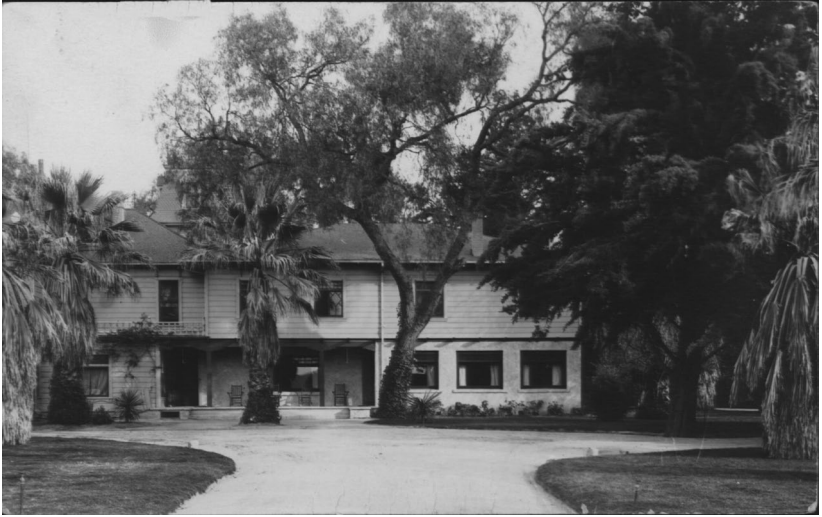
(Top) Same view only closer to the Inn showing drive approaching the front. (Courtesy of the Postcard Collection of Steve Lech)
